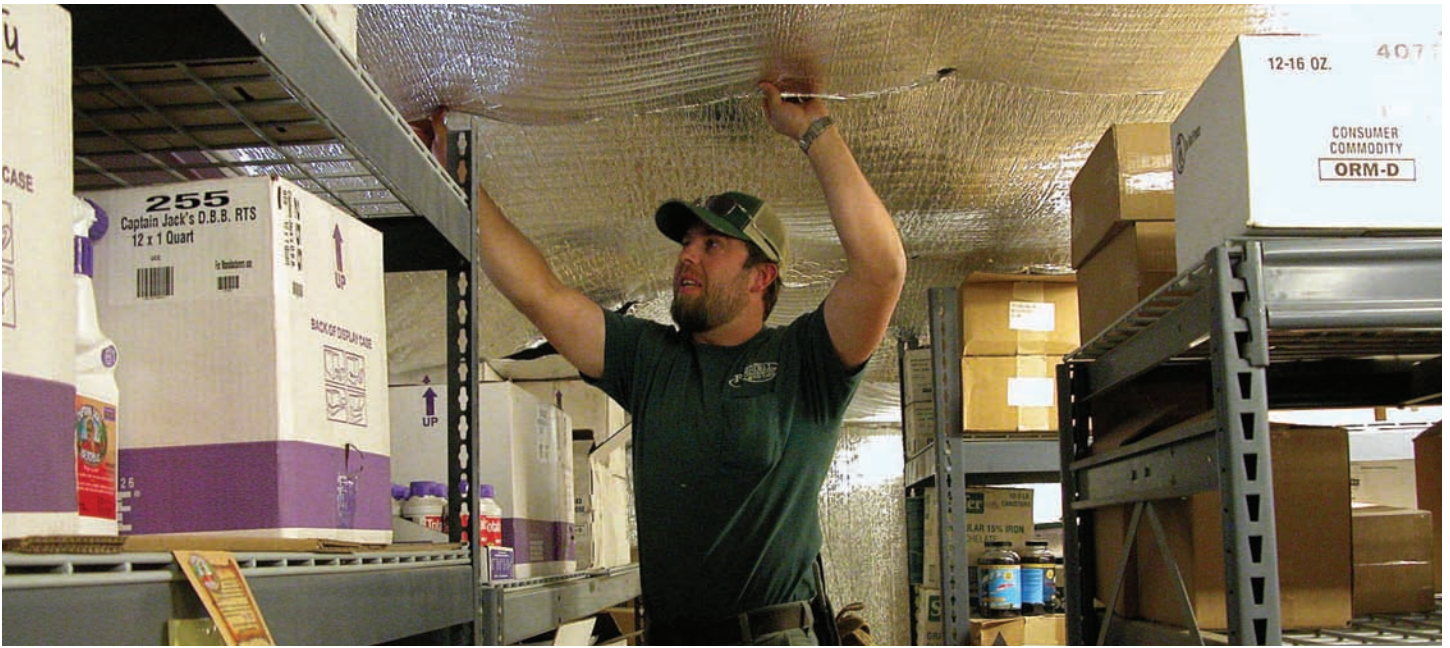
Rivendell General Manager Jared Kerst looks over the foil-lined reflective insulation that helps control temperature extremes in the metal-roofed product storeroom.
