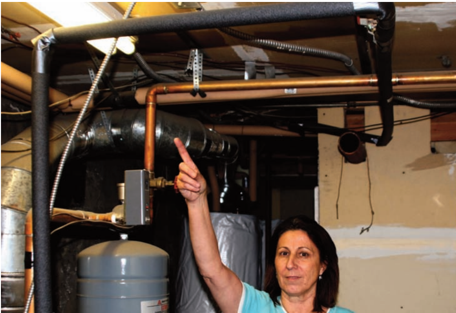
Left: Savage Land Co. office manager Joanie Hibdon shows the foam pipe insulation added to exposed hot water pipes in the basement. Right: Sally Brands with an insulated hot water pipe on the building's main level.
