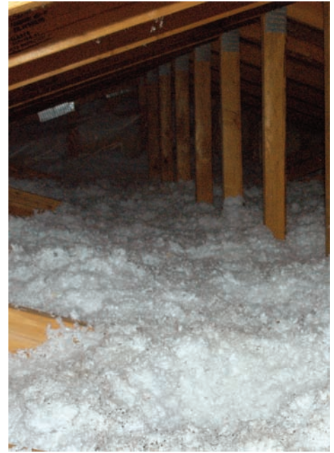
Right: Mittleider believes it's mostly the vast amount of new insulation blown into his attic that has cut his electricity bills.
